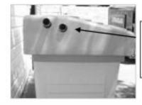
Cut holes with hole saw ½" larger than piping.
