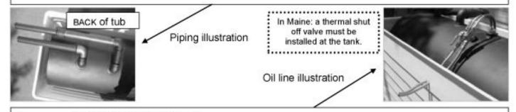
Refer to diagram above. Due to Limited access to the bottom of the tank, the oil lines CAN ONLY be pulled from the top of the tank.
